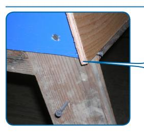
Cut a piece of plywood to fit the back of the coop, and attach it in the same manner as the side pieces. Be sure you leave an overhang for your roofing.
