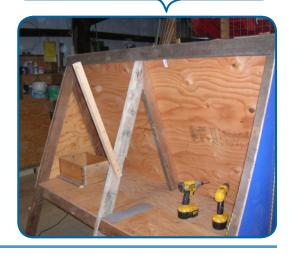
Attach the hinges to the 1x4 strip of wood that runs across the top of the door side of the coop, and cut a piece of plywood to use as the door.
