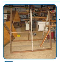
Right the frame of the coop, and square it corner to corner. Brace the frame corner to corner with scraps of 1x4, other lumber or plywood strips of material.
